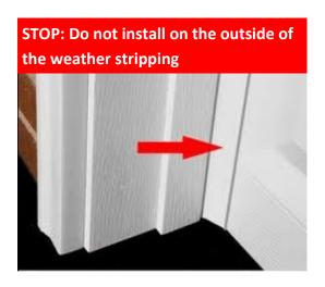
Install Rodent Shield on the inside of the weather strip as shown below.
